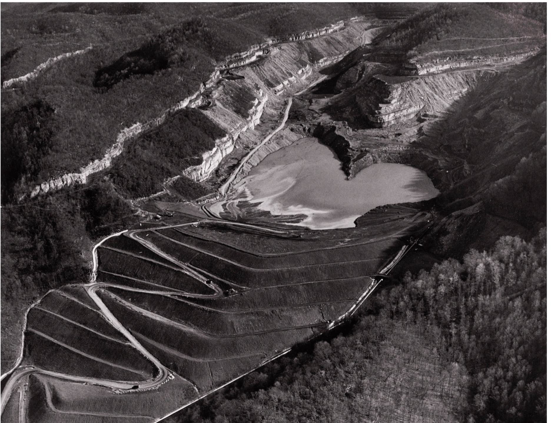
Brushy Fork Impoundment, Marfork Coal Co
